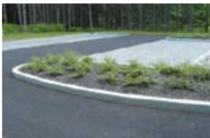
Rain Gardens (top) and porous asphalt are structural BMPs that infiltrate runoff.
